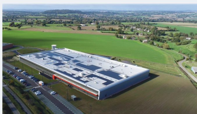
Aerial picture of THX One site – Thermocoax Normandy
